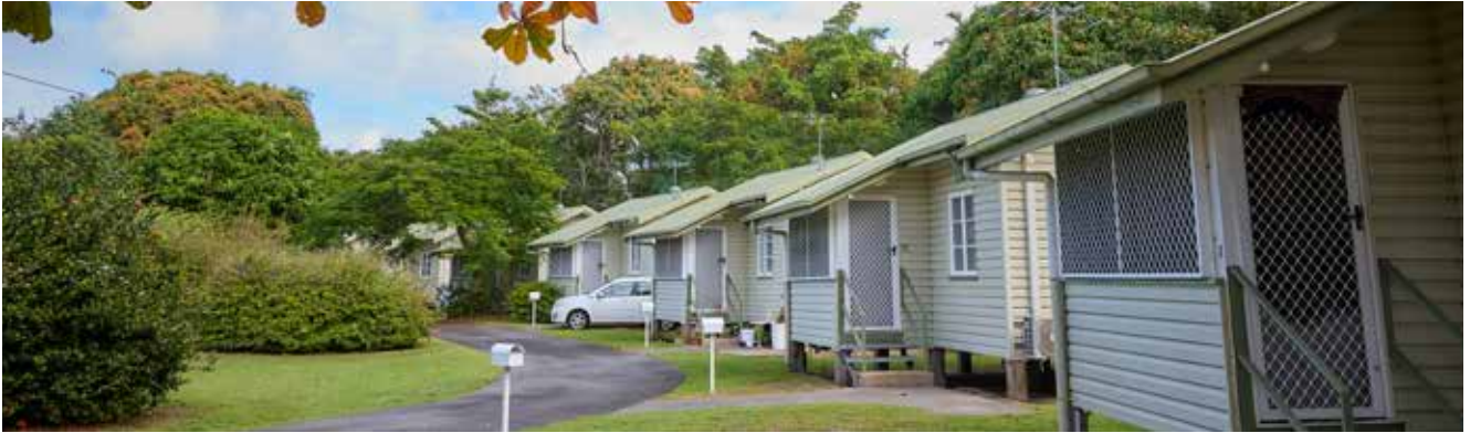
ABOVE: EIGHT INTERNALLY REFURBISHED COTTAGES.
